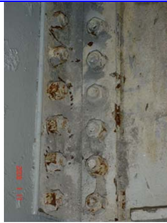
Figure 164. January 2008 rust (1/17/08) Source: Wood,
