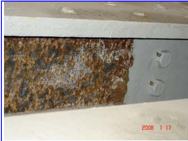
Figure 168. January 2008 rust (1/17/08) Source: Wood,
