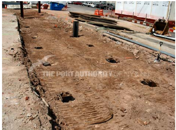
Figure 199. Rich dirt is used to cover the construction zone. (4/06)
