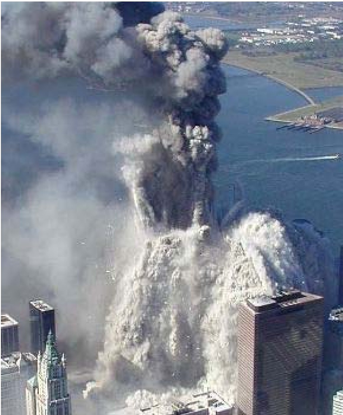
Figure 242. This does not look like a collapse to me. SAIC is complicit with the NIST report in calling this a collapse. That is fraud; they know better! (9/11/01)
