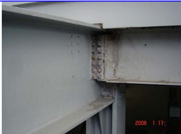
Figure 167. January 2008 rust (1/17/08) Source: Wood,
