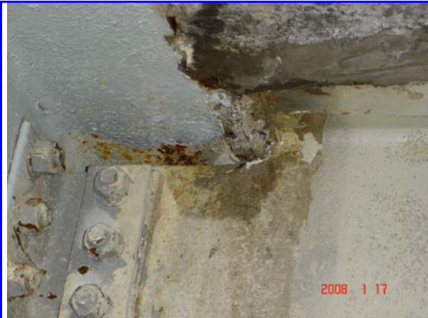
Figure 163. Hazardous degradation (1/17/08) Source: Wood,
