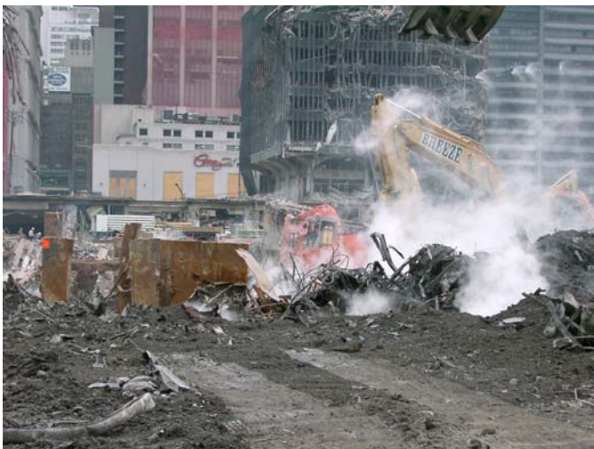
Figure 172. Fumes emerge from wet dirt. (10/31/01)
