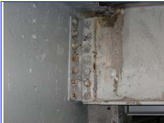
Figure 165. January 2008 rust (1/17/08) Source: Wood & Johnson,
