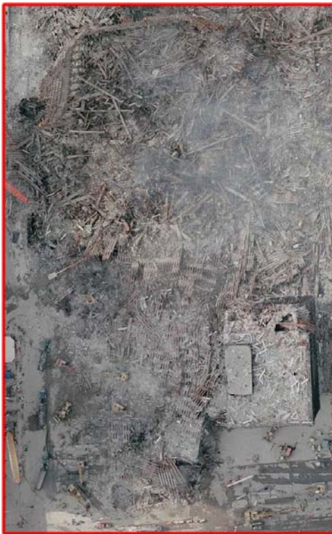
Figure 240. Figure 60. WTC4 footprint at the bottom, the remaining WTC4 north wing on the right, and the WTC2 footprint above. (9/23/01)
