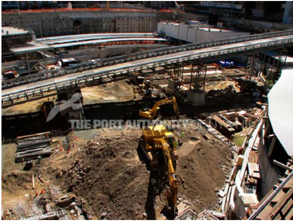
Figure 108. Dirt has been brought in to the west (big) bathtub. (9/07)
