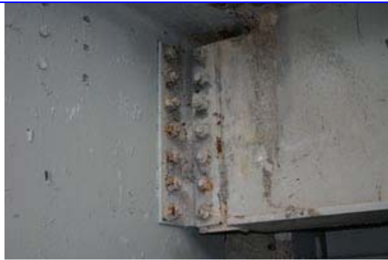
Figure 159. October 2007 rust (10/9/07) Source: Gerst & Wood,
