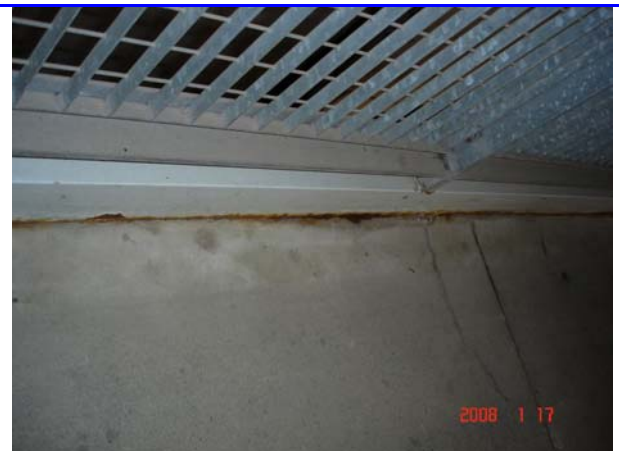
Figure 119. This is the temporary PATH train station below the area of former WTC5. (1/17/08) Source: Wood,
