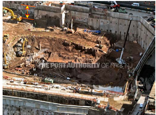
Figure 117. (October 2007) The dirt is about 2 stories below street level. (10/07)
