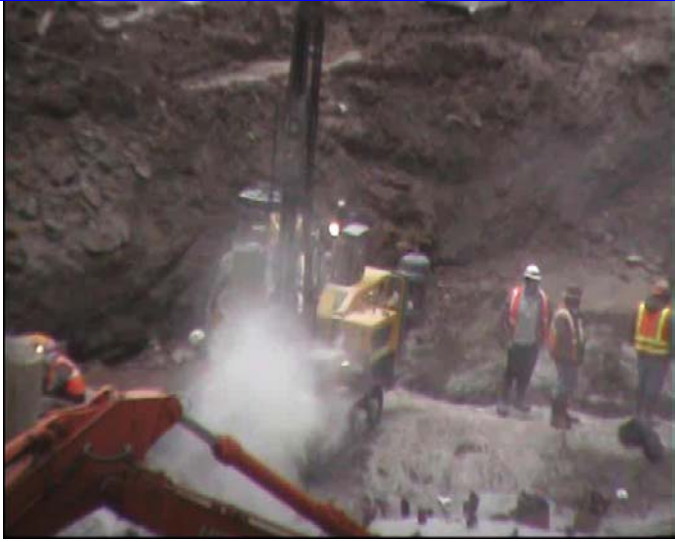
Figure 136. Digging stirs up fuming. (1/17/08) Source: Wood, Johnson,
