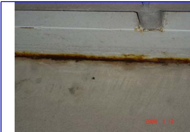
Figure 118. Extraordinary rust in the temporary PATH train station. (1/17/08) Source: Wood,
