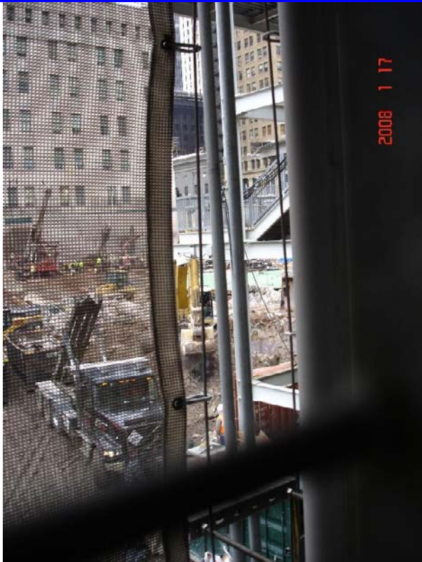
Figure 127. Moving dirt without fuming. (1/17/08) Source: Wood,
