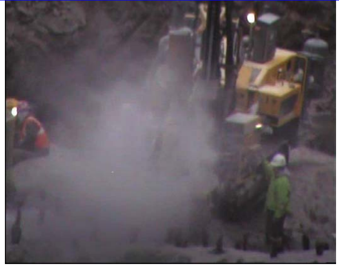
Figure 137. Digging stirs up fuming. (1/17/08) Source: Wood, Johnson,
