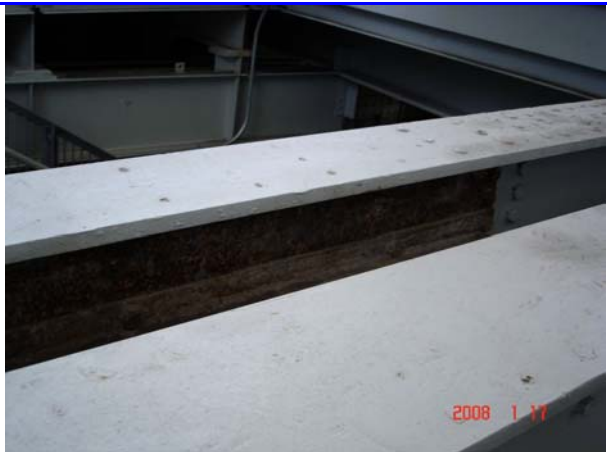
Figure 162. January 2008 rust (1/17/08) Source: Wood,
