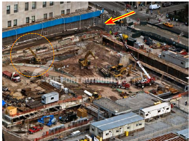
Figure 111 The dirt is lower than ground level. (10/07)
