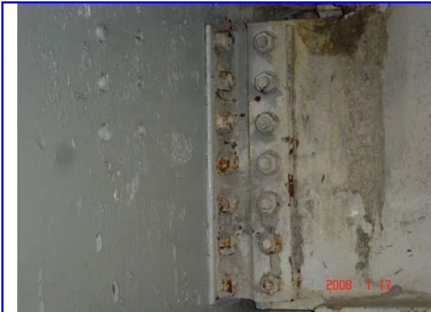
Figure 161. January 2008 rust (1/17/08) Source: Wood,
