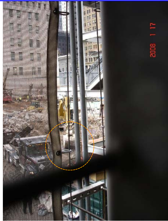
Figure 125. Power shovel scoops up dirt. (1/17/08) Source: Wood,
