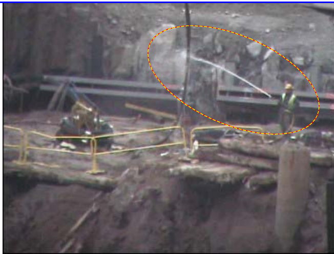
Figure 133. Hosing down a suspended cable at the WTC Site, 17 th Jan 2008. . (1/17/08) Source: Wood, Johnson,
