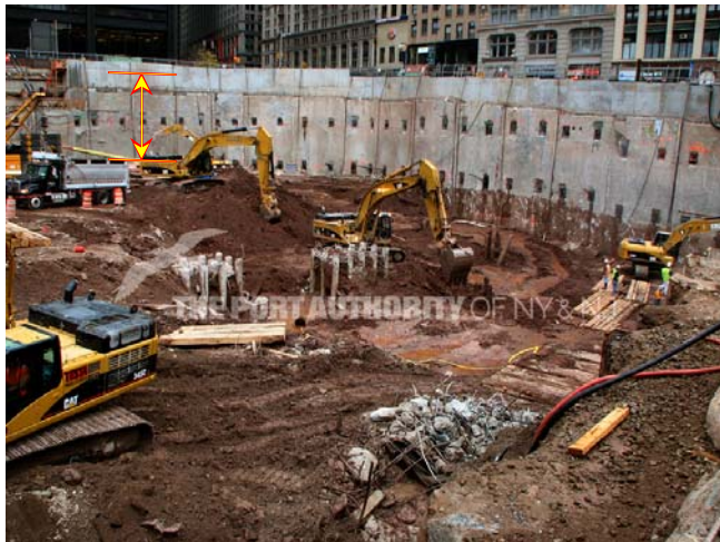
Figure 116. (October 2007) The dirt is about 2 stories below street level. (10/07)
