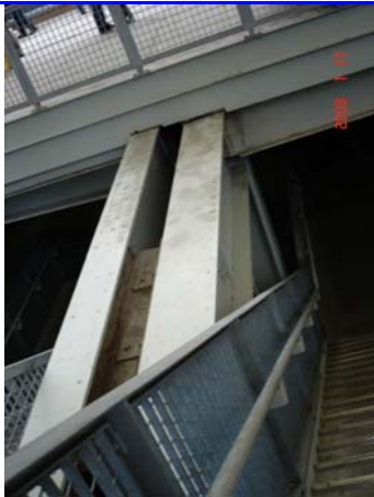
Figure 158. January 2008 rust (1/17/08) Source: Wood,
