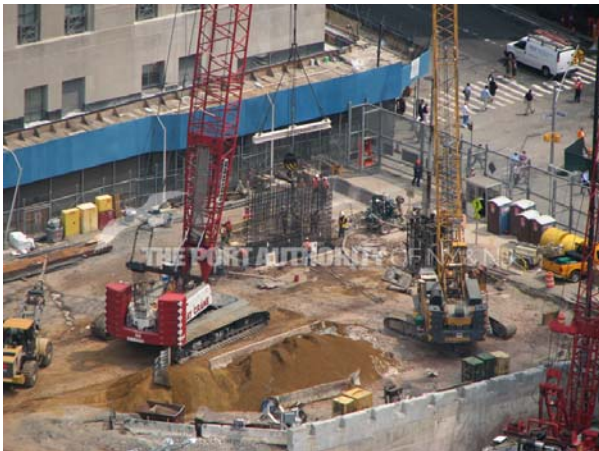
Figure 106. Dirt has been brought in to the west bathtub (August 2007). (8/07)
