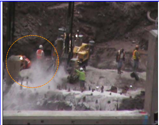
Figure 134. Digging stirs up fuming. (1/17/08) Source: Wood, Johnson,
