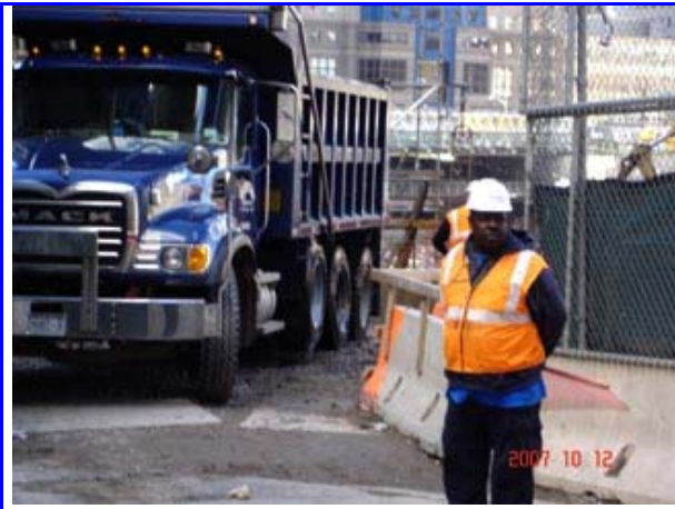
Figure 148. Guarding truck entrance/exit. (10/12/07) Source: Wood, Gerst,
