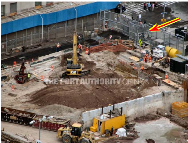
Figure 110 The dirt is higher than ground level. (10/07)
