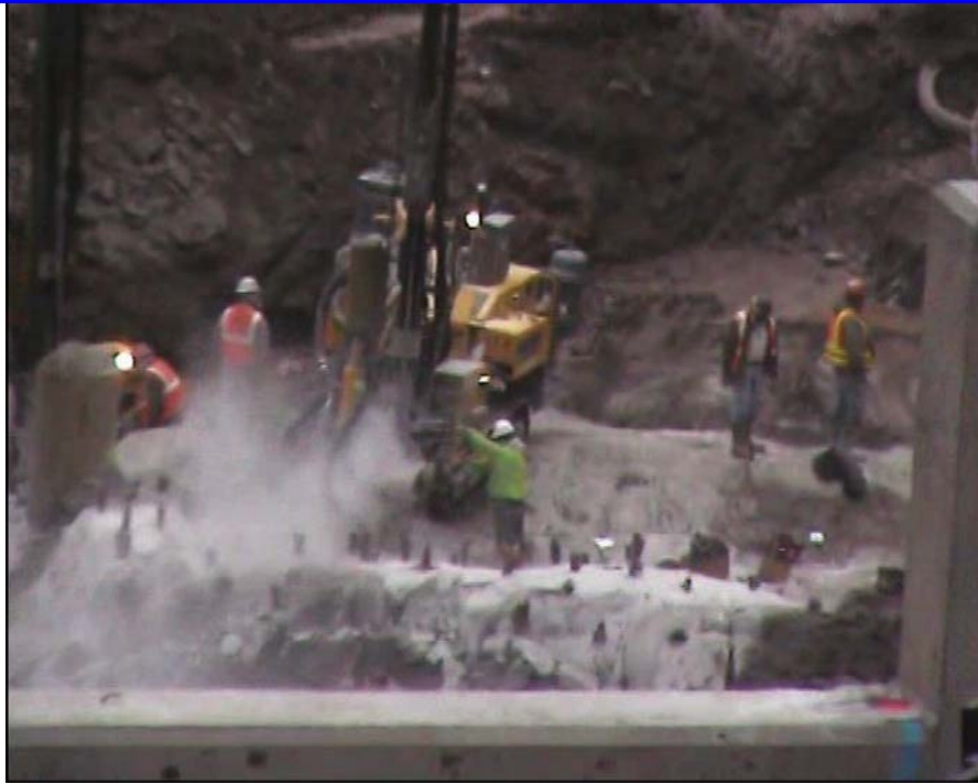
Figure 138. Digging stirs up fuming. (1/17/08) Source: Wood, Johnson,
