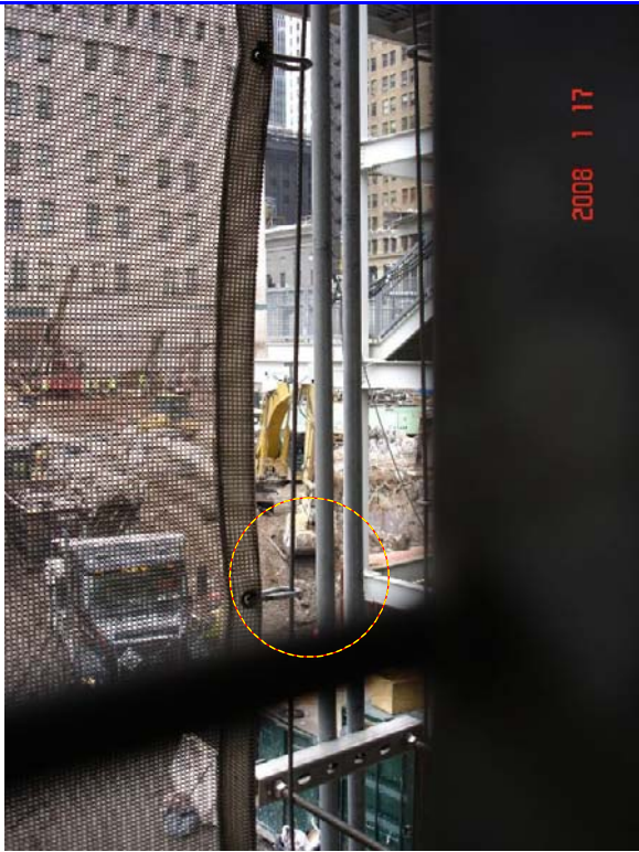
Figure 124. Power shovel pushes dirt around. (1/17/08) Source: Wood,
