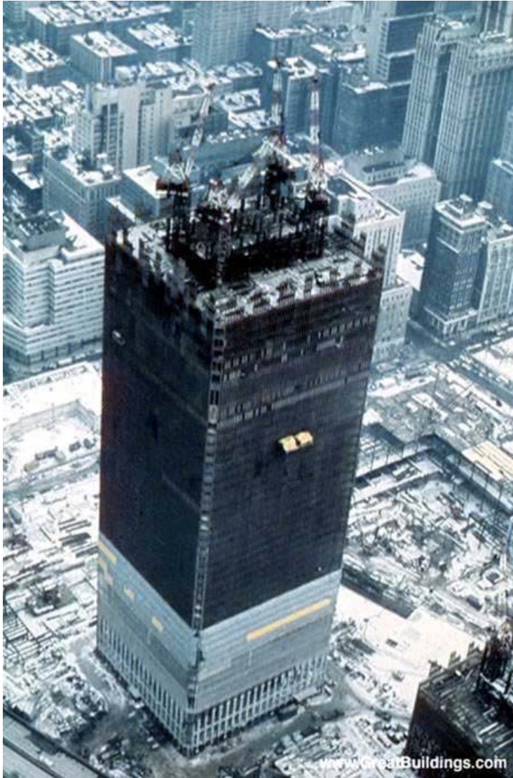
Steel-frame: Huge core (left) is an enormous heat sink. Notice workers standing on floor pan which is firmly attached to the interconnected core columns.
